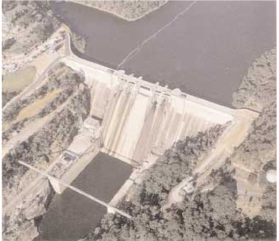
The raised and strengthened Warragamba Dam.
