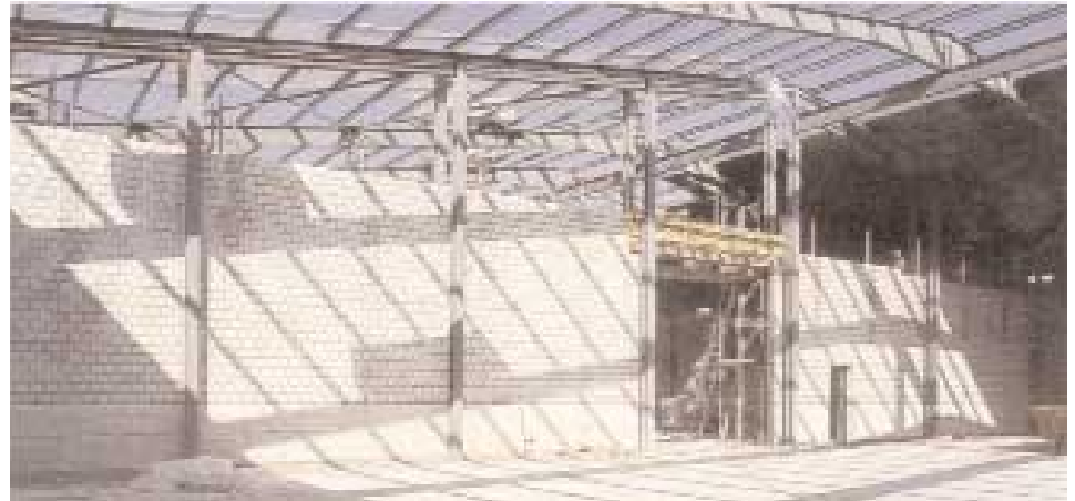
Post-tensioned fireproof factory wall under construction
