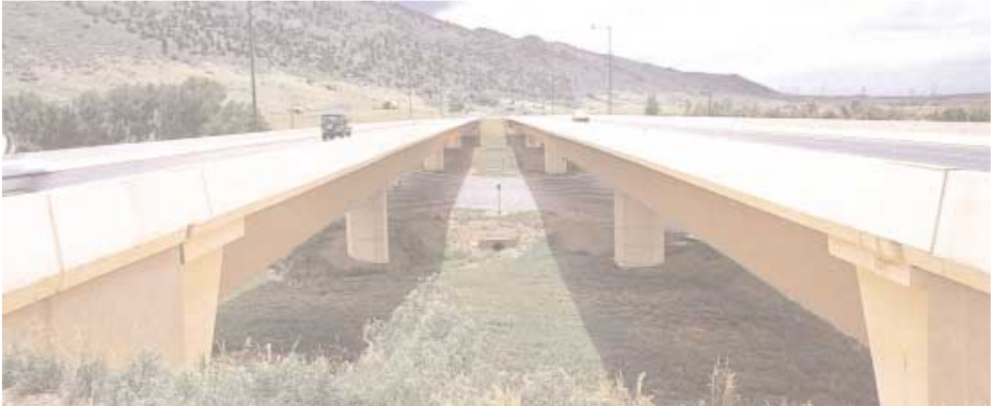
Cast-in-place, post-tensioned box girder structures have proven to be the most cost-effective solution for long-span Colorado bridges.
