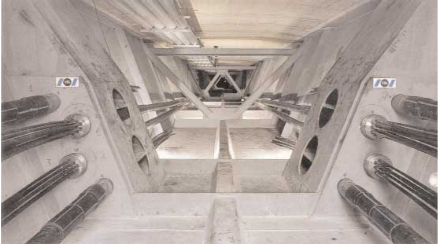
VSL's new external post-tensioning system utilizes individually greased and sheathed monostrands for increased corrosion protection and reduced tendon friction.
