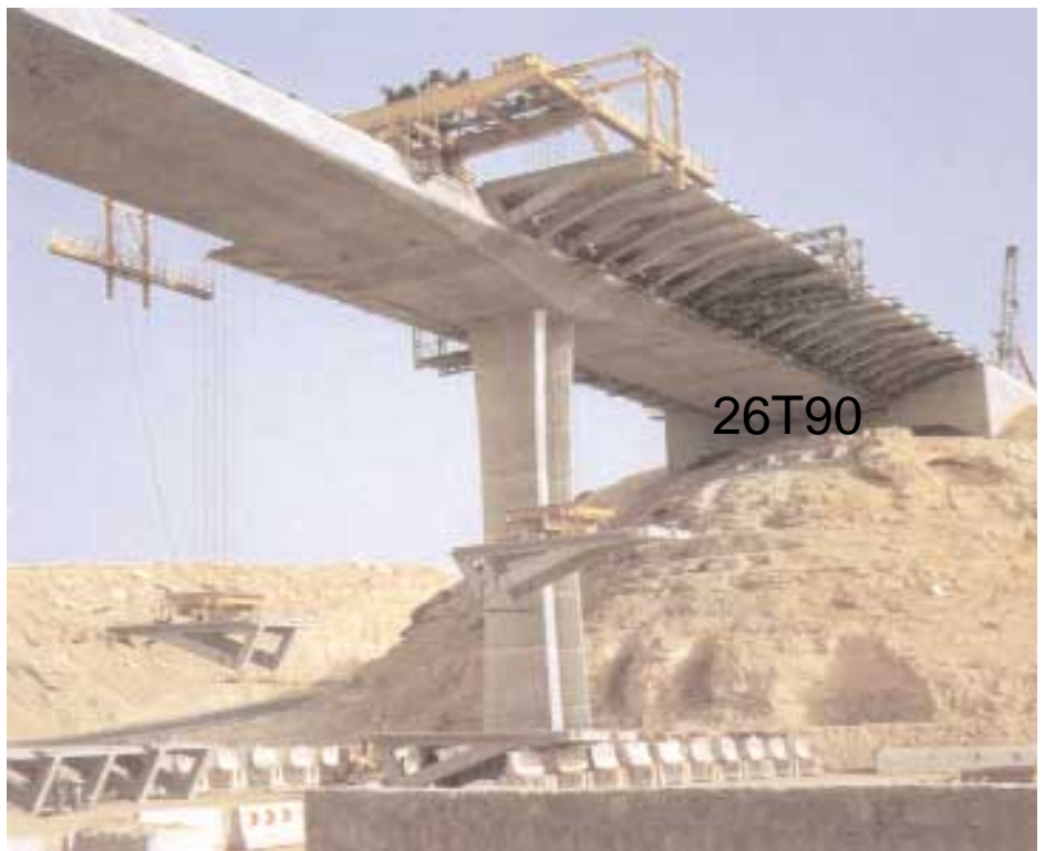
Lifting operation for precast side frames.
