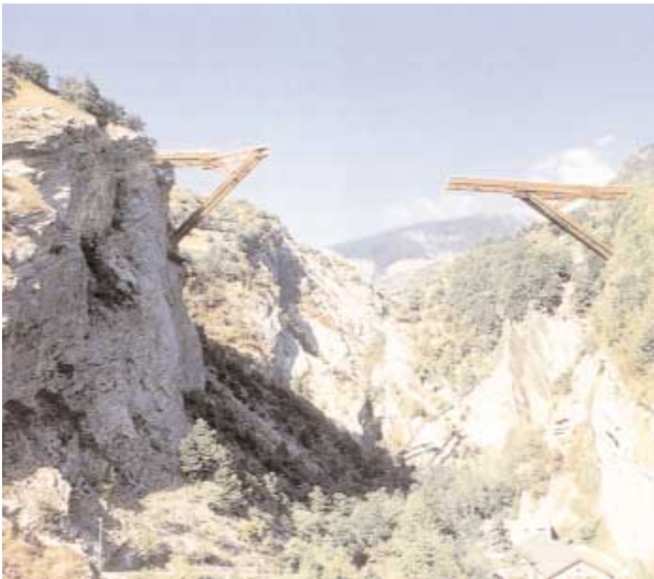
Heavy Lifting techniques feature in bridge construction.
