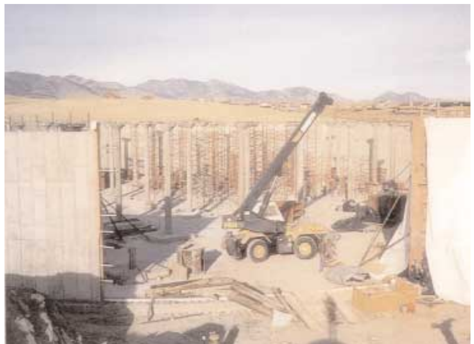
Colorado tank has post-tensioned floor, wall and roof.
