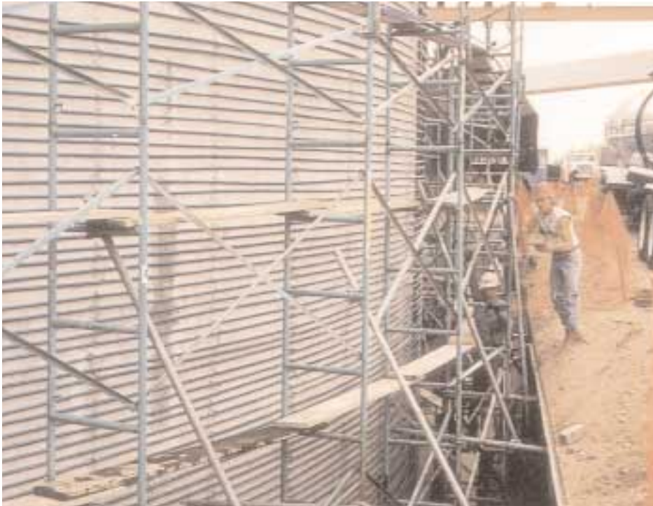
Tank life extended with VSL monostrand system.
