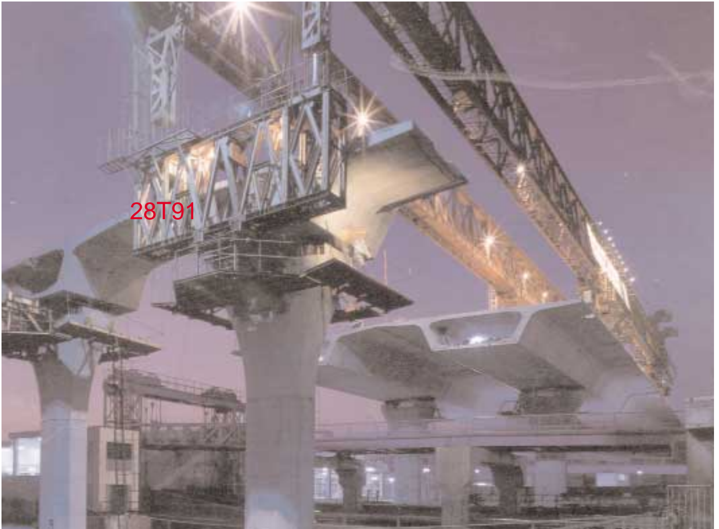
Post-tensioned free cantilever segments provide rapid construction progress.
