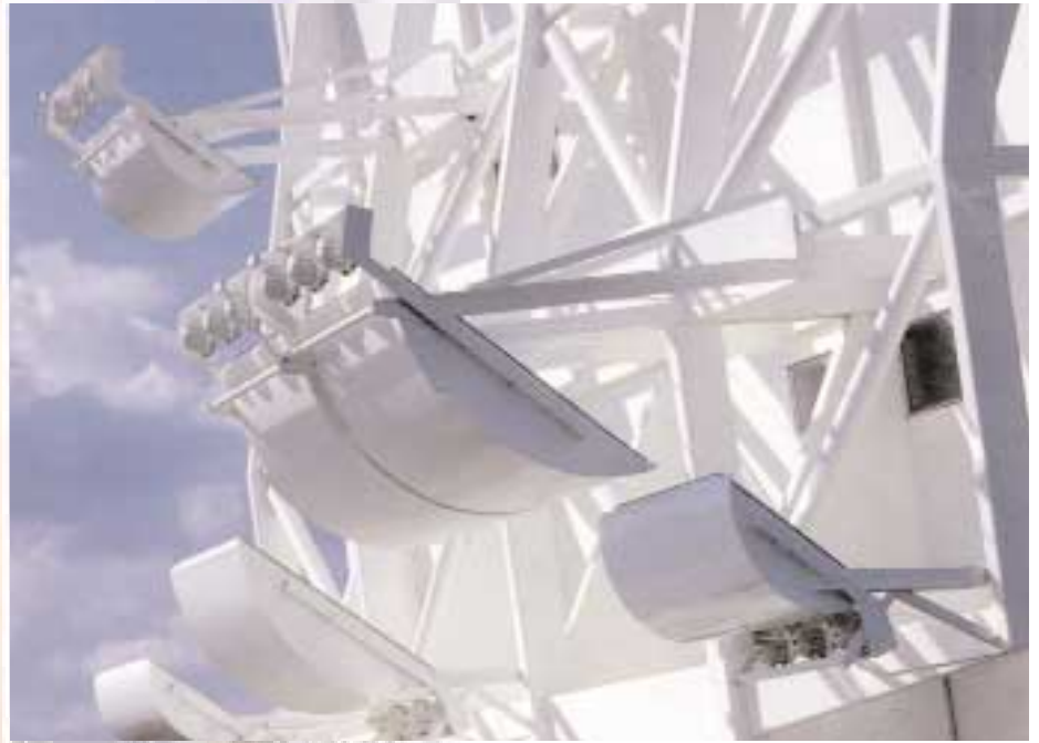
Mirrors attached to steel trusses at the rear of the rotating wall track the sun and reflect its light through the cut out names in the wall's granite.
