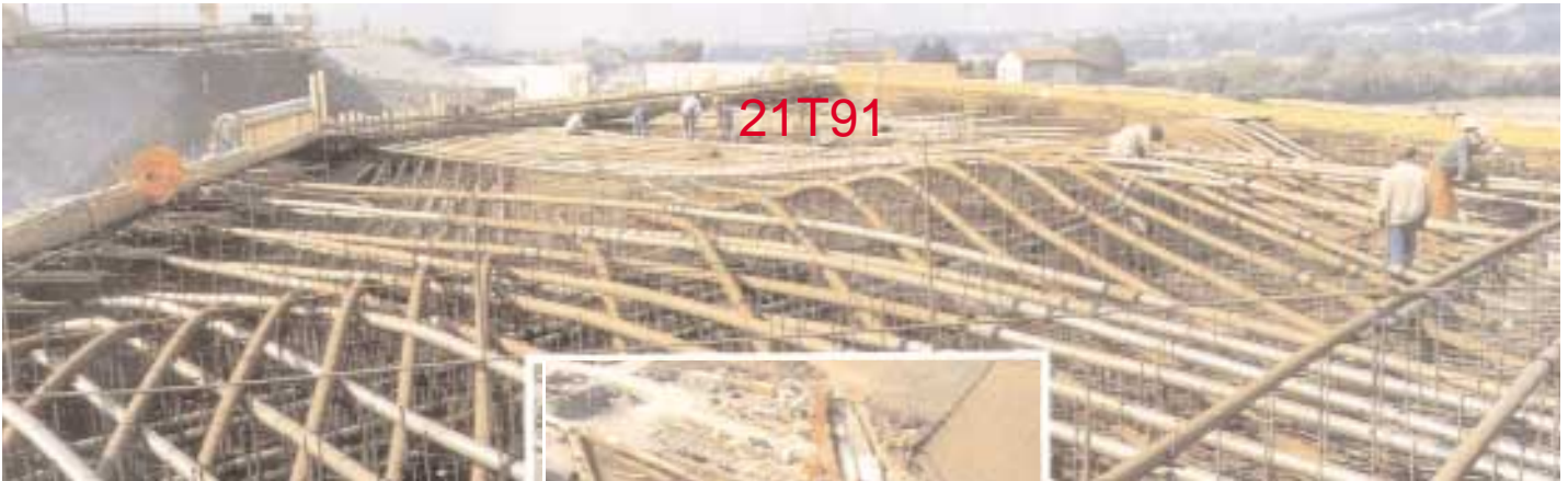
92 VSL E 5-31 tendons provide exceptional durability and structural integrity.
