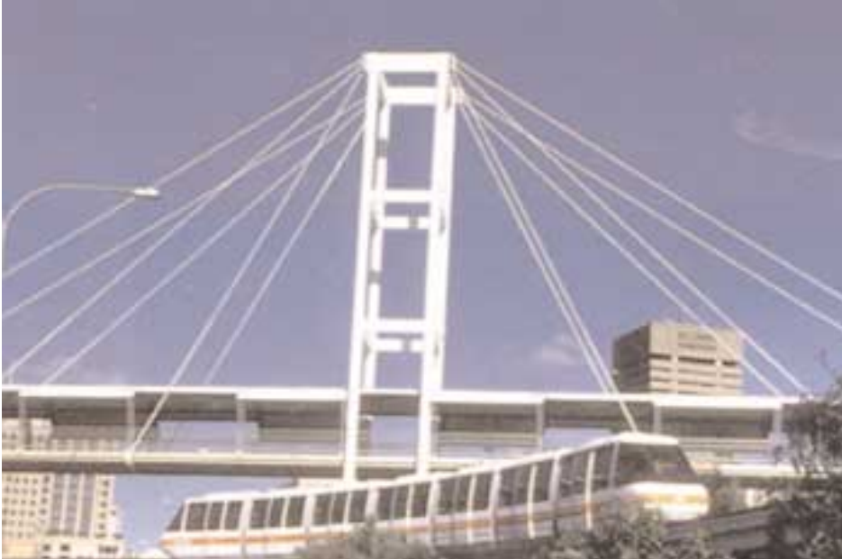
VSL Stressbar-stayed bridges are now in service at University of Western Sydney and the Darling Harbour complex.
