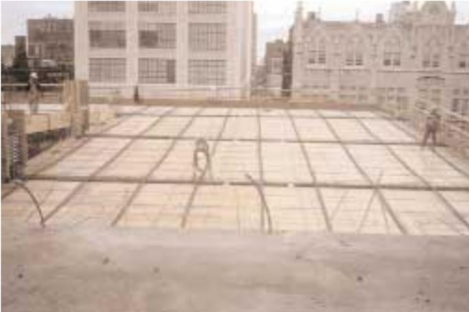
Installation of PT-PLUS flat duct
