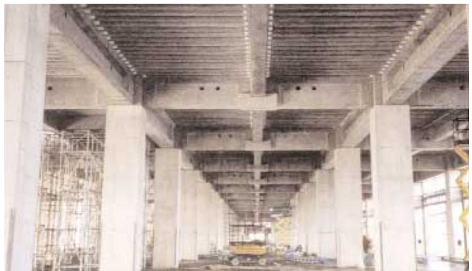
Precast concrete members are used for the 2nd and 3rd floors.
