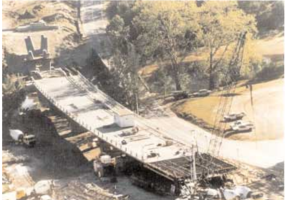
Casting bed and existing timber bridge in background
