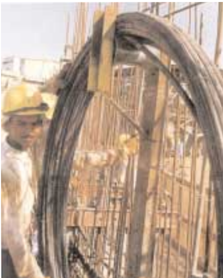
Reeled monostrands being installed during slipforming
