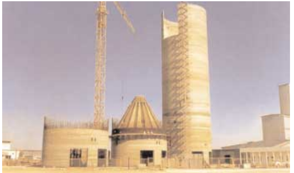
Slipforming in progress on Clinker Silo
