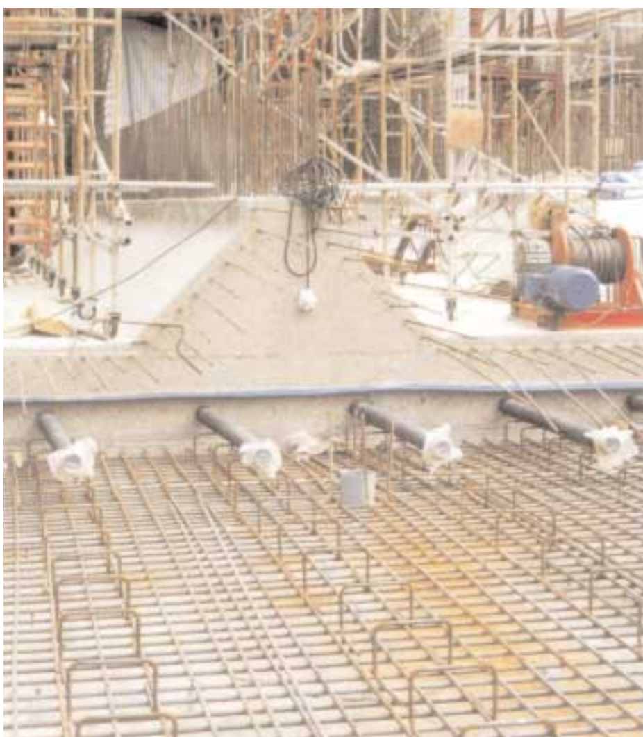
Construction Joint Base Slab
