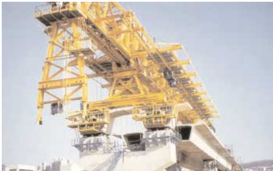
Span-by-span erection using one overhead truss covering two box lines simultaneously
