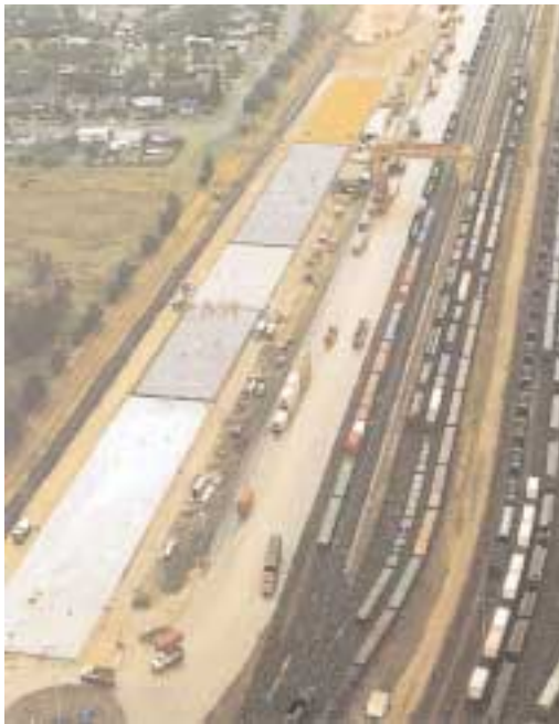
Post-Tensioning was the chosen solution for 1200 m of container pavement
