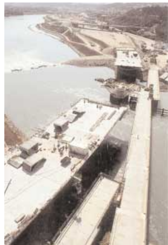
The BPNL viaduct over the Rhone river
