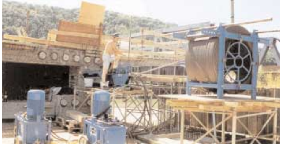
Pushing of the 193 m long tendons
