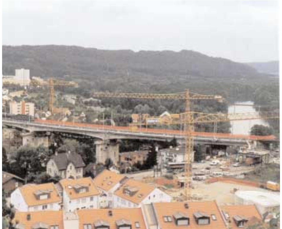
The railway bridge over the Aare river.
