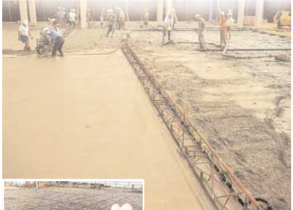
Post-tensioning of 42,000 m 2 of slab on grade greatly reduces jointing in the slab
