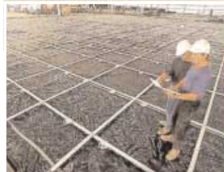
Post-tensioning of 42,000 m 2 of slab on grade greatly reduces jointing in the slab
